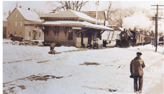
Boston & Maine Railroad Sta, Fitch Street
